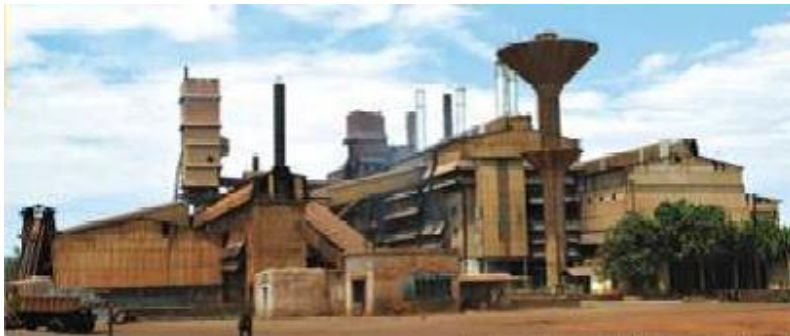
Ferro Chrome Plant at Garividi
