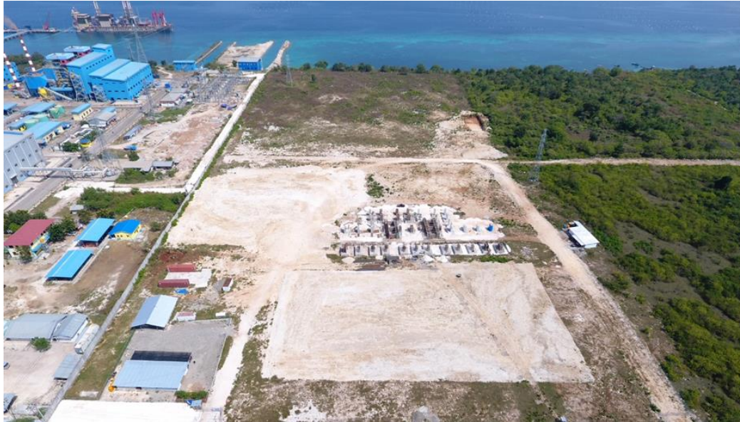
Figures 3 - Aerial overview of the Kupang Smelting Hub Facility site highlighting close proximity to power station (top left)
