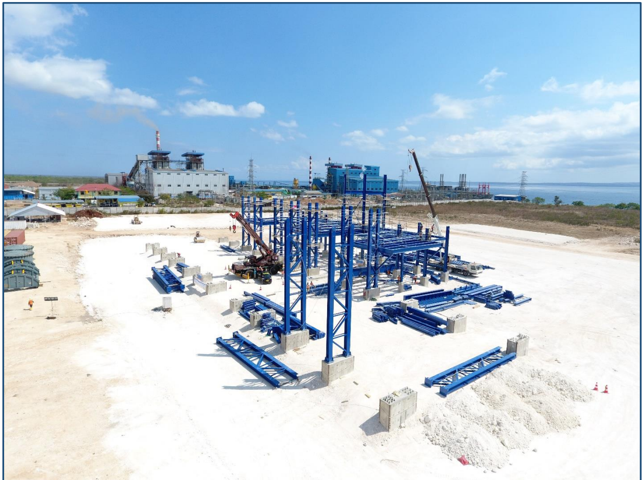
Figure 1: Construction progress at Gulf's Kupang Smelting Facility.
