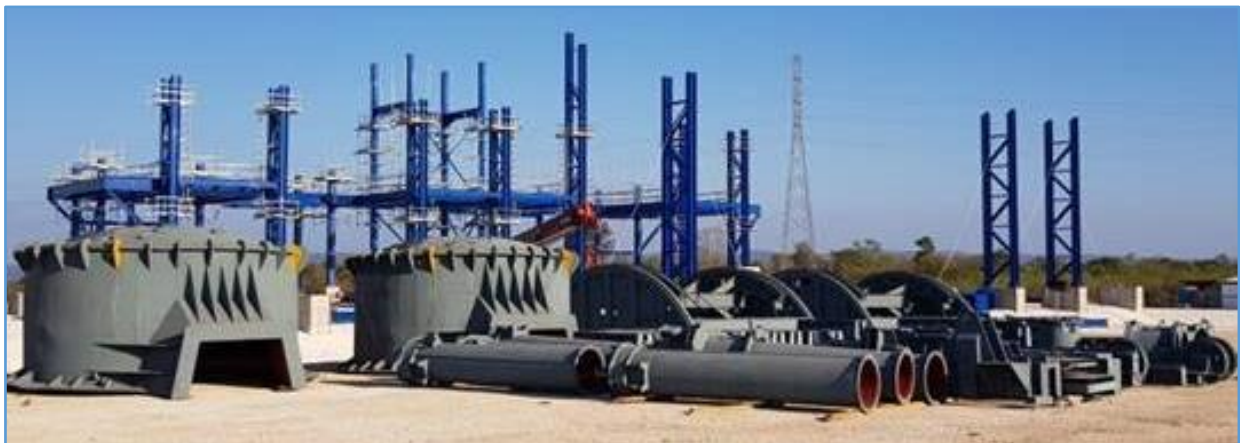
Figure 1: Construction progress at Gulf's Kupang Smelting Facility
