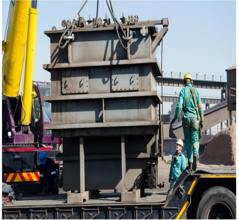
Figure 1 and 2: Furnace transformer transported from Transalloy to sub-contractors for refurbishment
