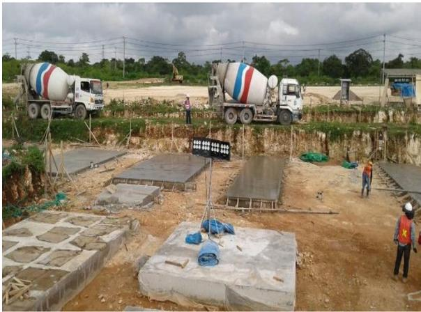
**Figure 2: Concrete slabs being poured on site**
