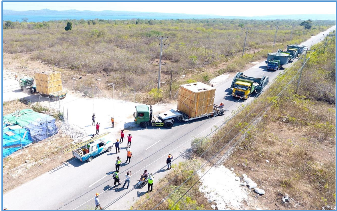
Figure 2 The furnaces arriving on site after transportation from the nearby Tenau Port, Kupang
